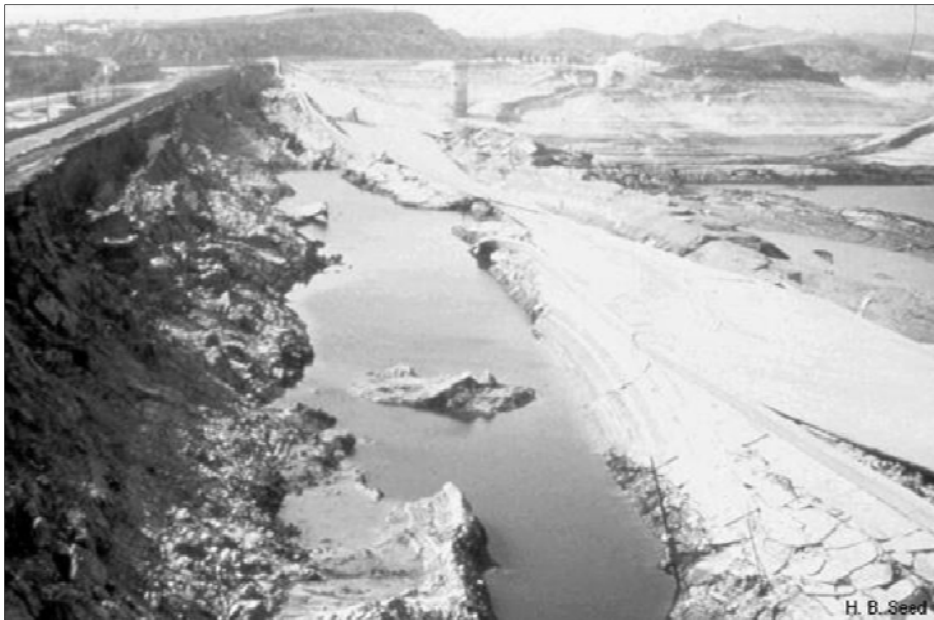
Figure 3. Lower San Fernando Dam after the 1971 earthquake.
