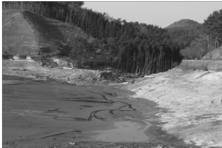
Figure 4. Fujinuma Dam after Tohoku earthquake of 11 March 2011.
