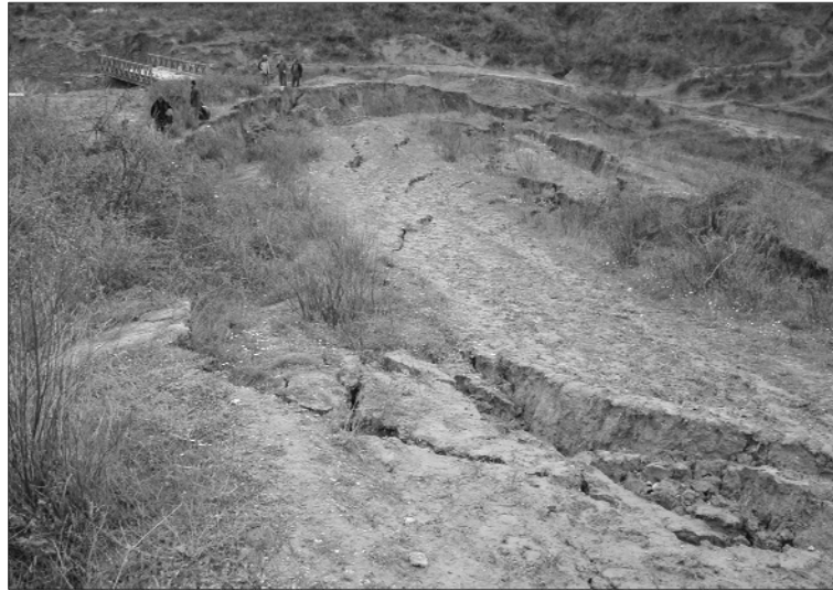
Figure 1. Sharredushk Dam in Albania after earthquake of 18 March 2009.
